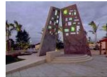
Cast concrete performance space, internally lit glass panels Height approx 6m Location – Carindale Shopping Centre, QLD
