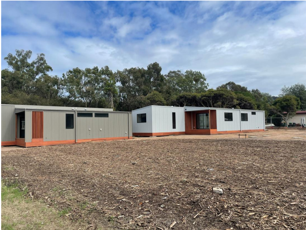
On site and finished
