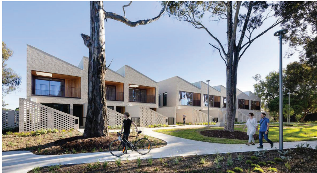
Precedent for a well designed precinct with market, social and affordable townhouses, within a tenure blind model: Tarakan Street Housing , by NH Architecture + Bird de la Couer.
