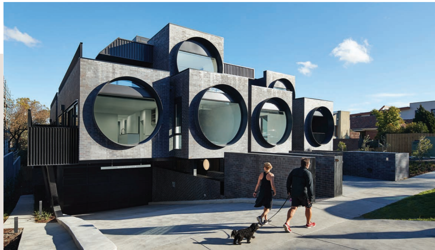
Cirqua, East Ivanhoe, by BKK Architects (photo: Peter Bennetts): Medium-density apartments which reference the suburban residential context, with a striking, engaging street frontage.
