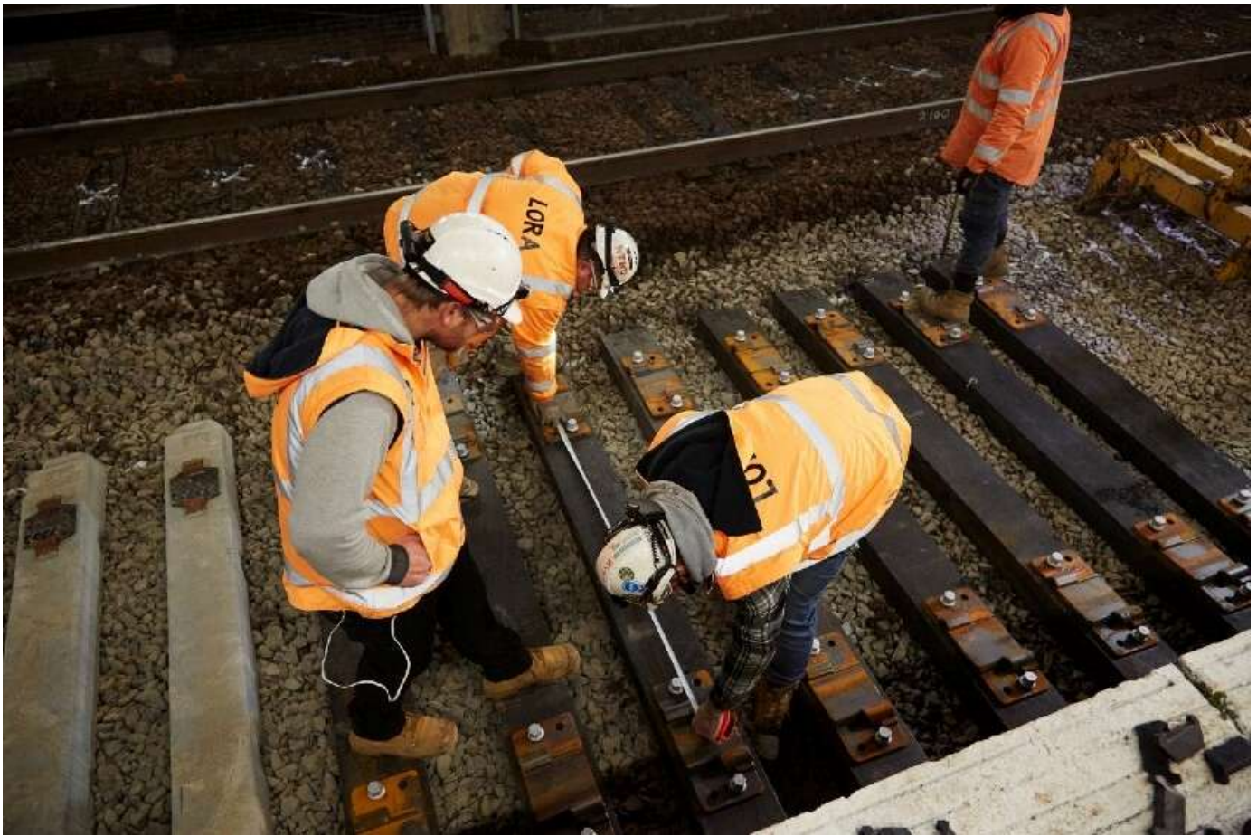
Laying Duratrack sleepers at the Richmond Station trial 2019
