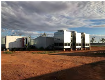
Thargomindah Water Cooling Project.
