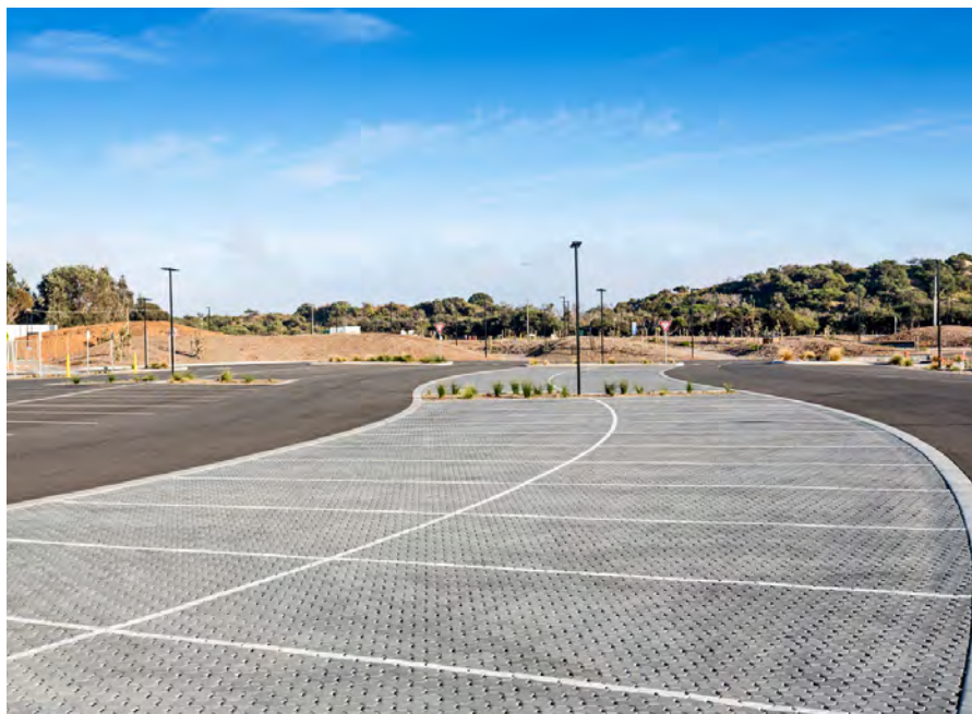
Figure 10 A completed PICP system on Phillip Island in Victoria, which allows for rainfall and runoff infiltration through small openings between individual paving units.
