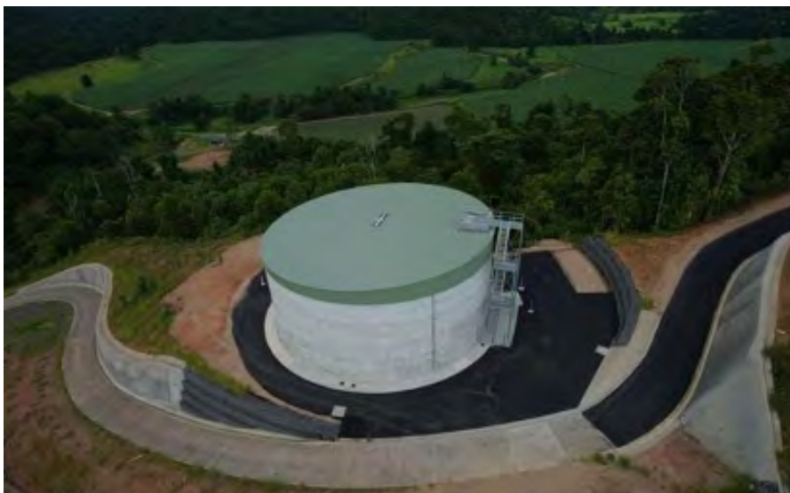
Nyleta Hill Reservoir – Completed.
