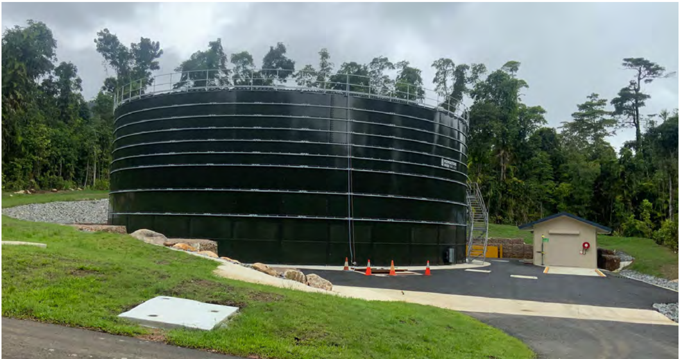
Completed Bulgun Creek Intake Reservoir.
