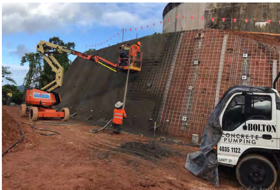
Bank stabilisation works adjacent to existing reservoir.
