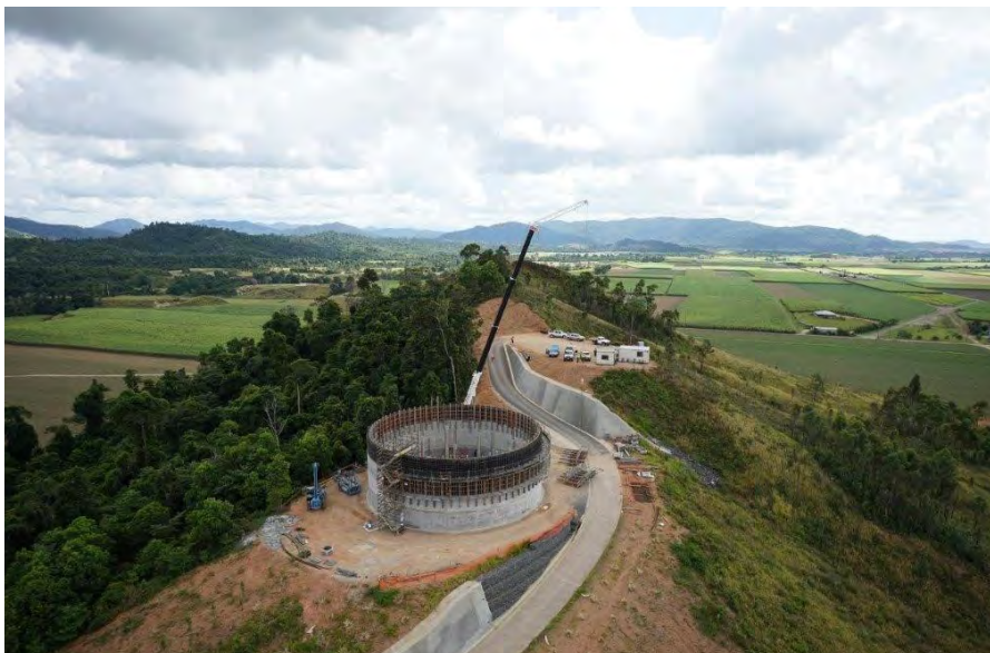
3.3 ML Nyleta Hill reservoir under construction.
