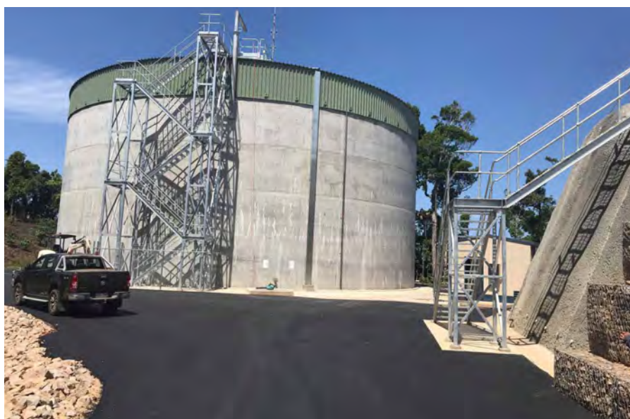
Completed Wheatleys Hill Reservoir.
