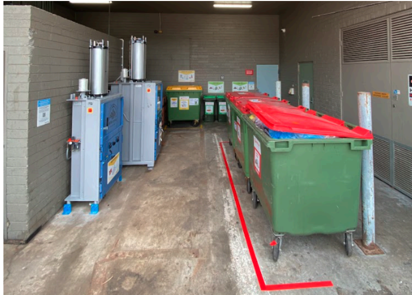
Image 1: Installation of shared bins within an enclosure operated by a central managing body, streams include: cardboard, soft plastic, mixed recycling, FOGO and general waste. Pictured: Mornington Peninsula Shire
