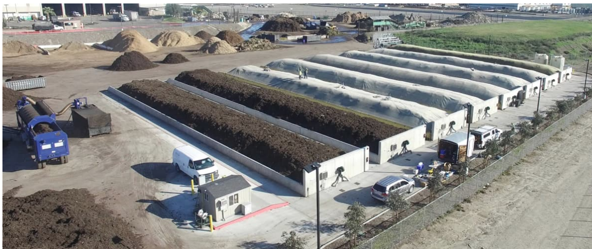
Figure 3.4: Covered static aerated composting
