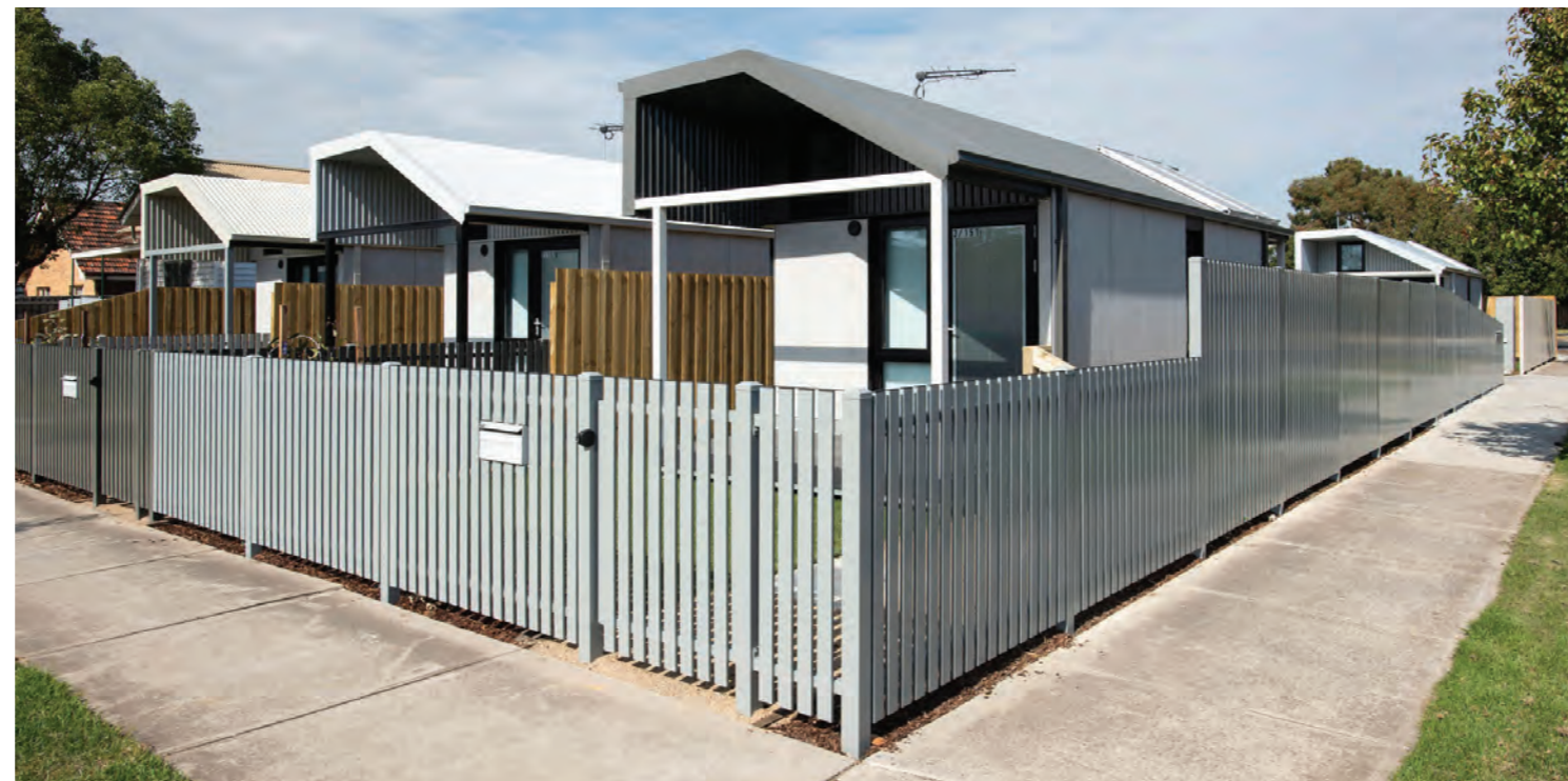
Portable housing units, Maidstone, for Launch Housing (source: Schored Projects).
