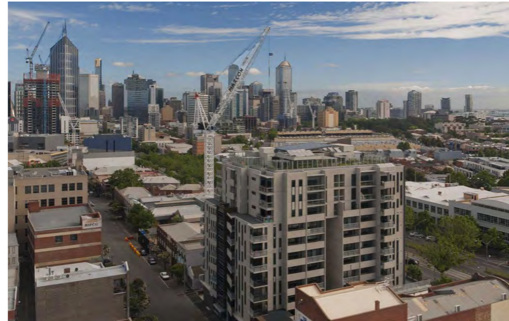
Common Ground, Stoll Architects (2010), 660 Elizabeth Street, Melbourne. Housing to support needs of people who have experienced long term homelessness. https://stollarchitecture.com.au/projects/common-ground-660-elizabeth-street-2/
